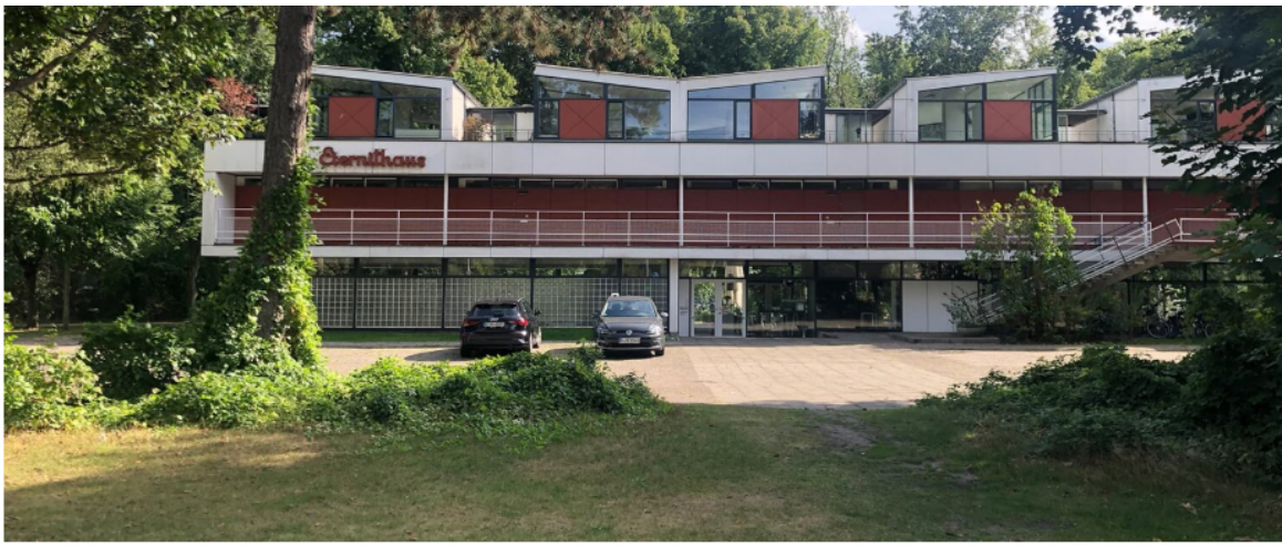
cement house. Photo: Tina Roeder.
